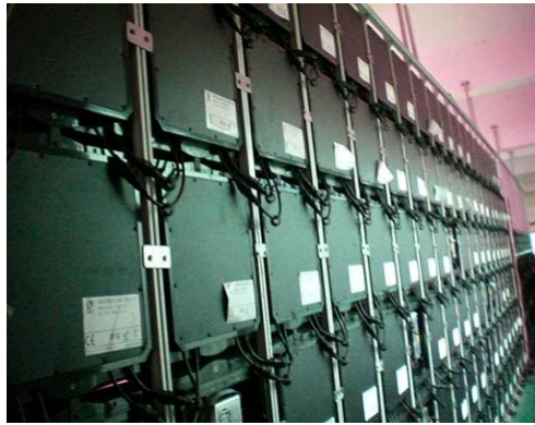
Modules installed on a chassis
