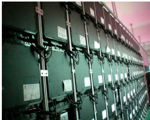
Modules installed on a chassis
