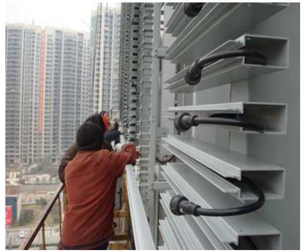
A Led wall is being installed on a facade and showing transparency (Model EVLW-37H)
