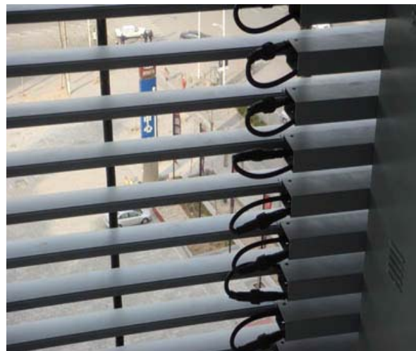
A Led wall is being installed on a facade and showing transparency (Model EVLW-37H)
